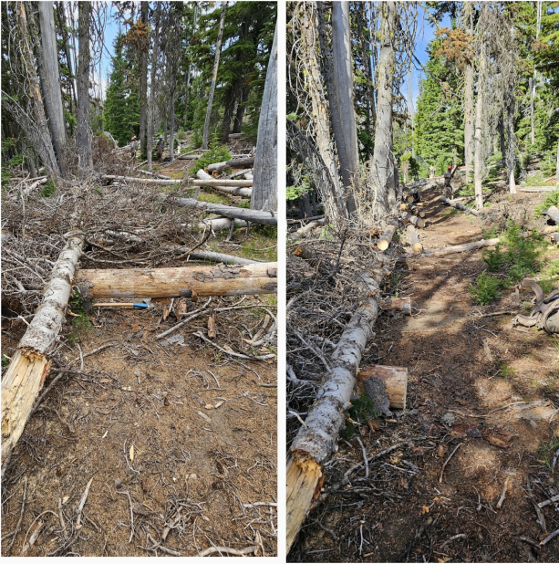
Crib Walls at Newberry National Volcanic Monument
